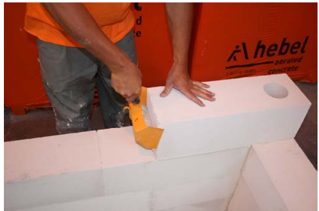
Figure 5D.12: Laying Hebel AAC cored-block
