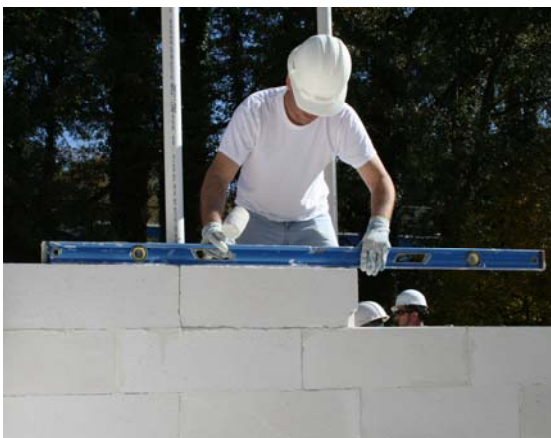
Figure 5D.10: Checking alignment and level of wall
