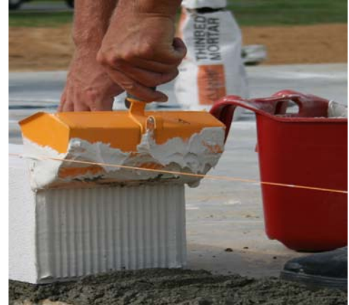
Figure 5D.3: Applying Hebel AAC thin-bed mortar to vertical joint with notched trowel
