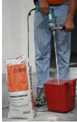
Figure 5D. 2: Mixing thin-bed mortar
