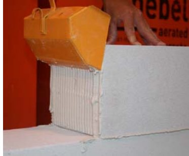
Figure 5D.6: Applying thin-bed mortar on all vertical joints
