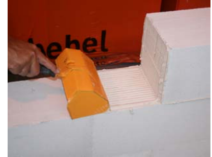
Figure 5D.7: Applying thin-bed mortar on horizontal joints
