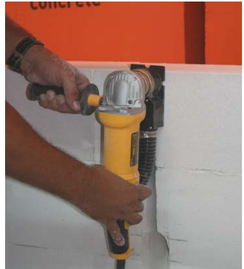
Figure 5D.13: Cutting chases into AAC wall
