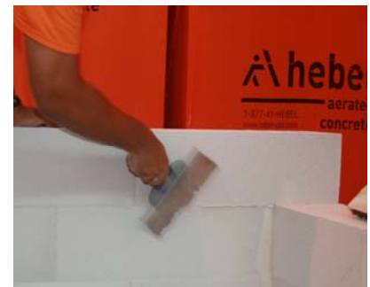
Figure 5D.9: Removing spilled mortar from joints
