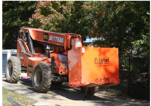
Figure 5D.1: Transporting Hebel AAC block
