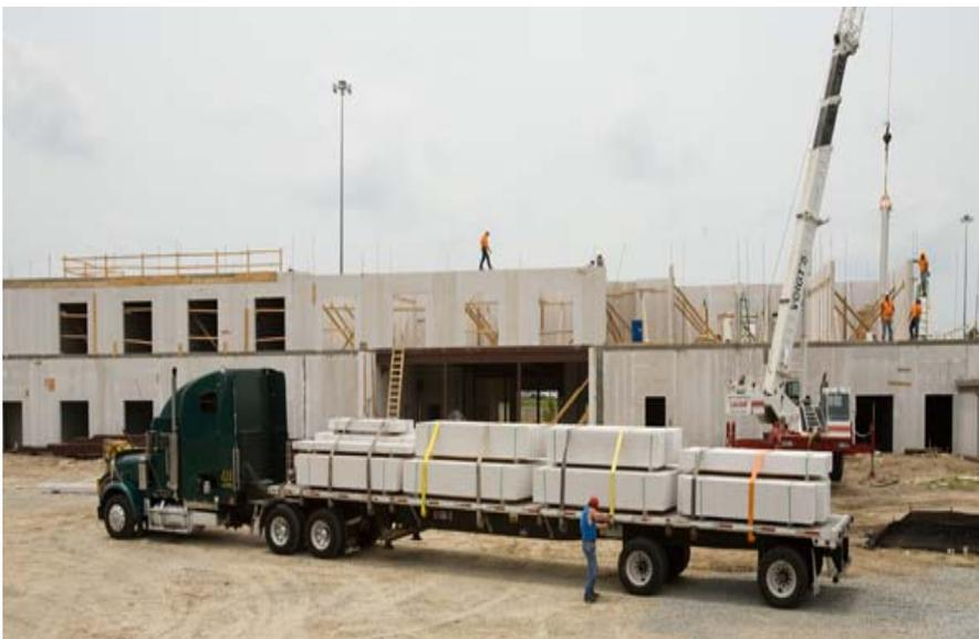
Figure 1.10: Hebel AAC Delivery to Project Site
